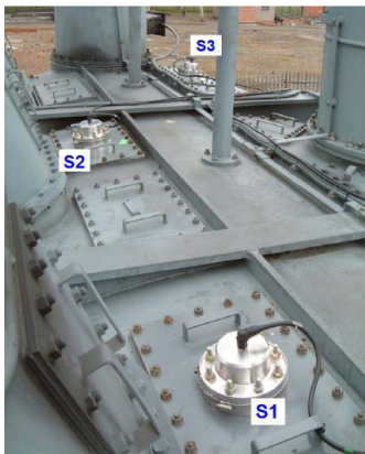
Figure 3: Sensor retrofit example and installation procedure
